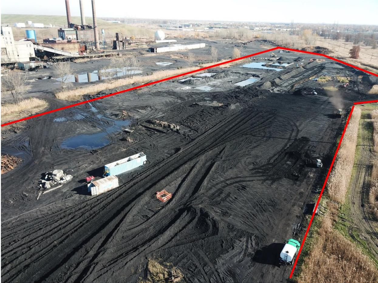
*Photo 4-8: Looking Northeast across the Coal Yards during regrading and prior to establishing stormwater BMPs.*
