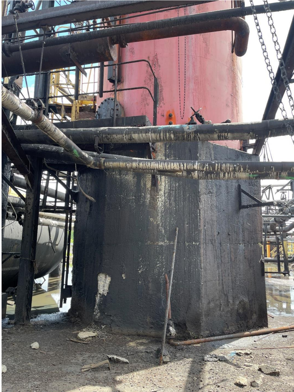
Photograph 2: Concrete Base, No Visible Tar Collection Sump
