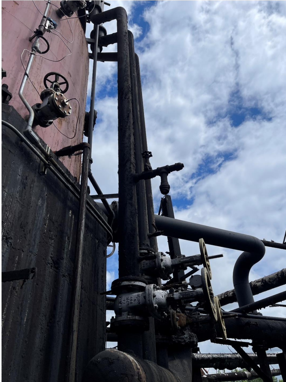
Photograph 7: 3-inch to 4-inch lines off southeast side of primary cooler, all lines tie into the north pipe rack running to the Pump House.
